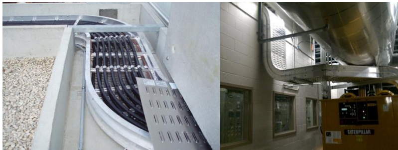
Figure 5 – Cablebus installed outdoors (left) and indoors (right)
